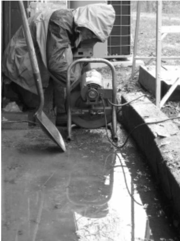
Chris Kohlstaedt cleans out the drain pipe.
