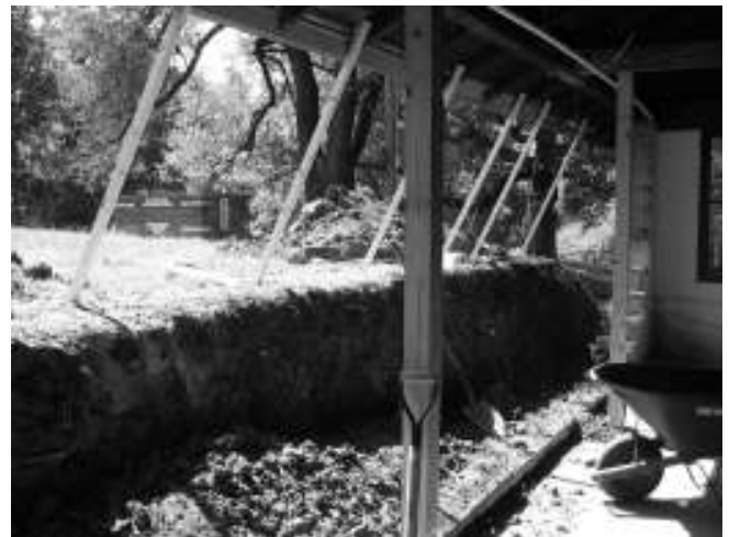
Chalet wall was demolished and much dirt removed.
